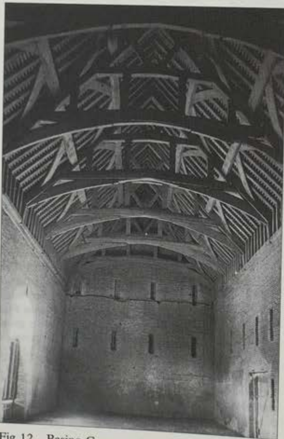
Fig 12 Basing Grange – The Great Barn, interior.
