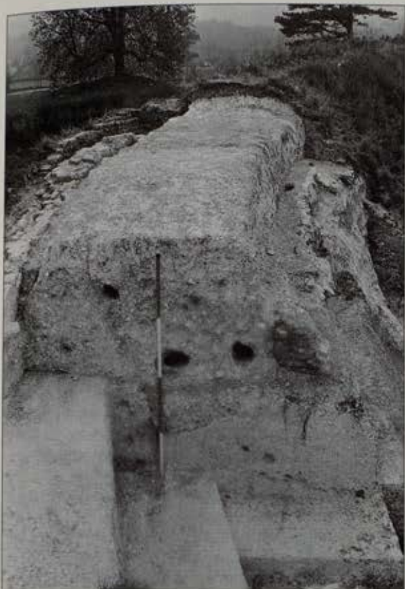
Fig 70 View of the Citadel Bank section from the east. The old ground surface is visible just below the midpoint of the ranging pole; the adjacent voids are rabbit burrows.
