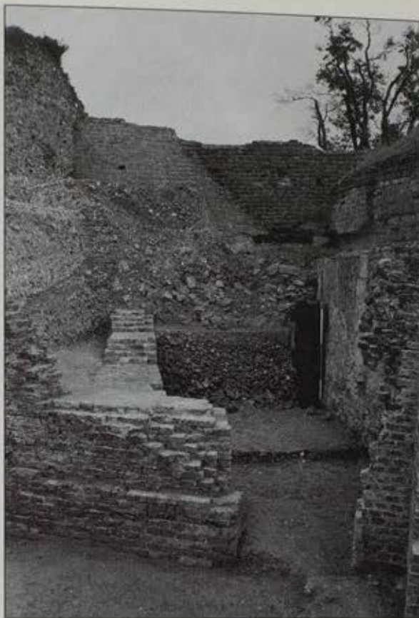
Fig 75 View from the interior showing the successive narrowing of the west end of the Postern Gate passage.
