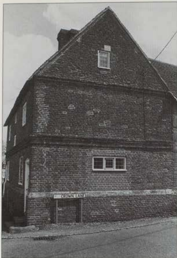
Fig 10 17th century house on the corner of The Street and Crown Lane, built with material taken from Basing House ruins.
