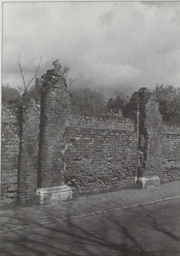
Fig 13 View from the south of one of the two blocked gateways which originally led to the late 17th century mansion.
